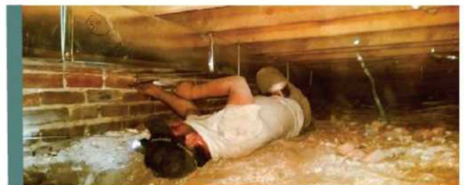
Cramped conditions in crawlspace
