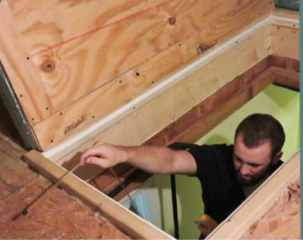
Pre-entry survey before entering attic
