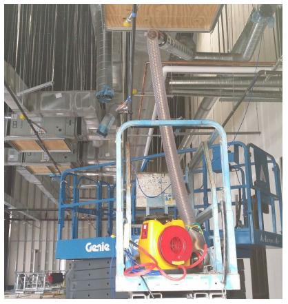
Figure 10 Model 400 Blower set up to test ducts prior to installation of the Flow Plug that is needed to measure flow.
